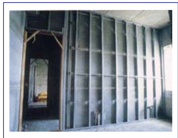
▲ 輕鋼架隔間牆施工中案例
